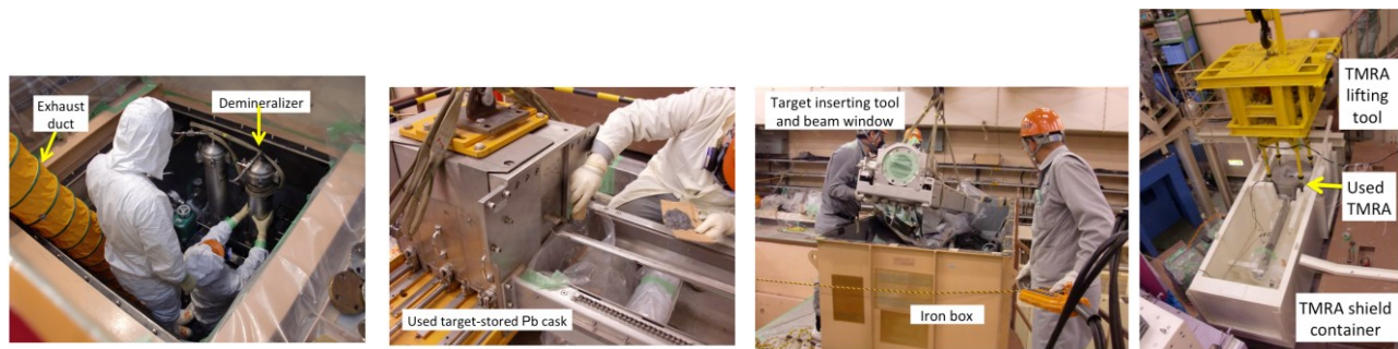
(1) Removing demineralizer and filter. (2) Separating the target moving device from Pb cask. (3) Storing the target moving device into iron box. (4) Carrying down TMRA to container.
