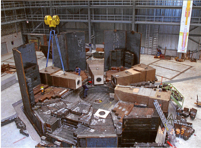
Figure 4 The SINQ target block during construction.
